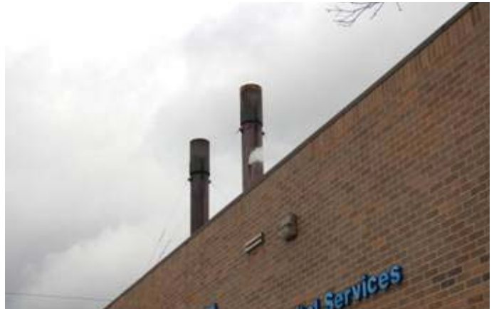
A steady loss of flash steam (see stack above) from the boiler feed tank posed another costly problem for plant operators.
