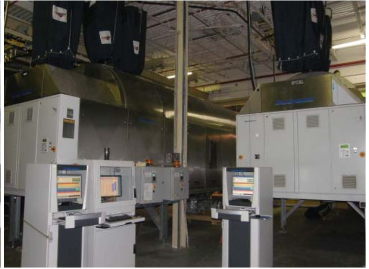
A look at the plant's two new Kannegiesser tunnel washers with an automated loading system that has largely eliminated the use of carts on the wash floor.
