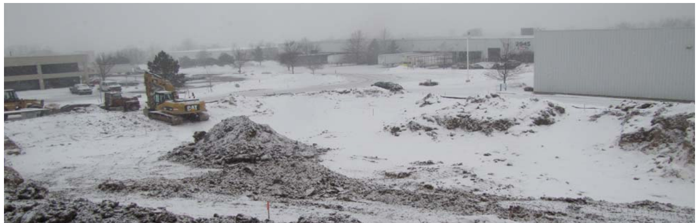
This is Michigan ... construction continues under any conditions!
