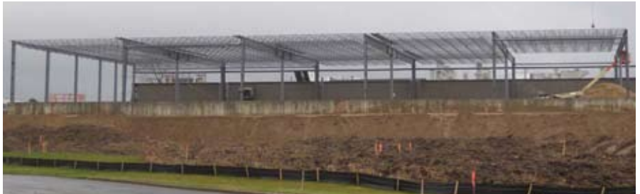
Above is a view of the frame of the building expansion.
