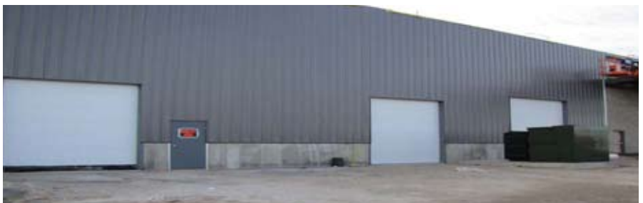
Here is a view of the completed expansion, including new electrical service transformers.
